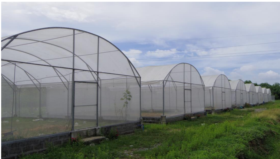
Figure 3. Greenhouses at PSU Sta. Maria Campus
